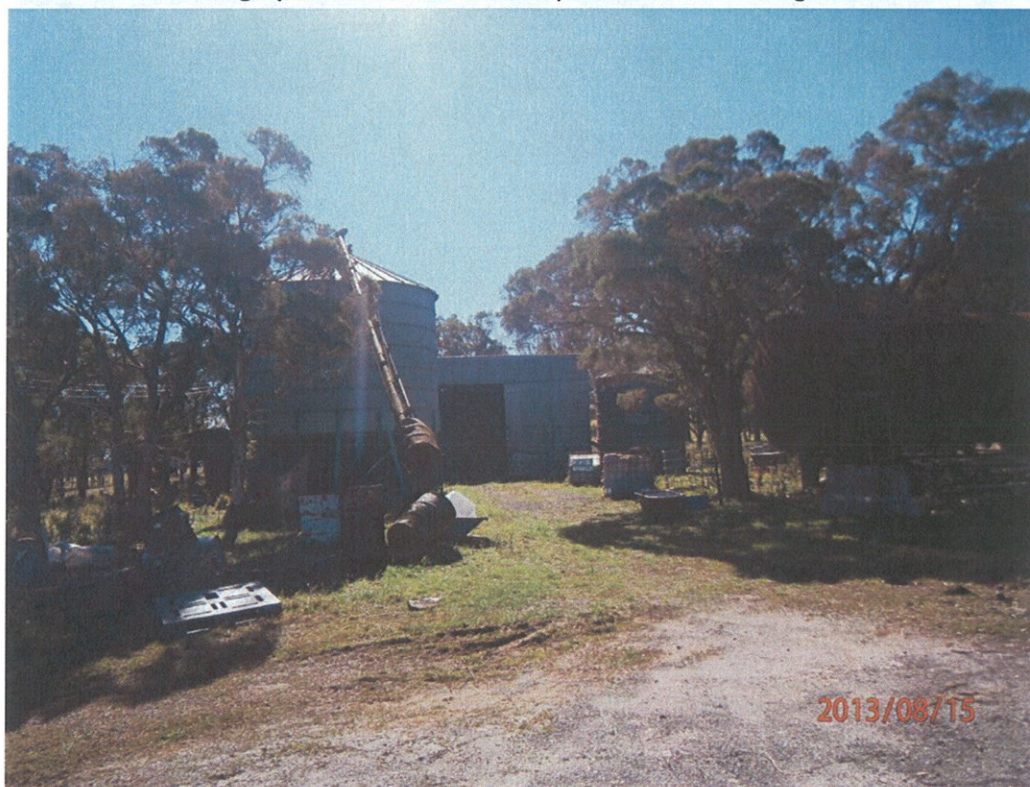
Photograph 2 – View of the work area of Lot 201 looking north
